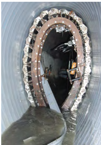
Sewer rehabilitation with the SPR™ spiral-wound pipe technology is no problem under live flow conditions.
