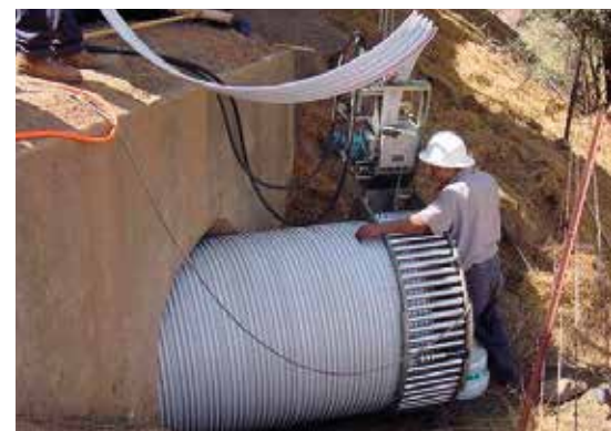
The winding machine winds the PVC profile to form a liner
