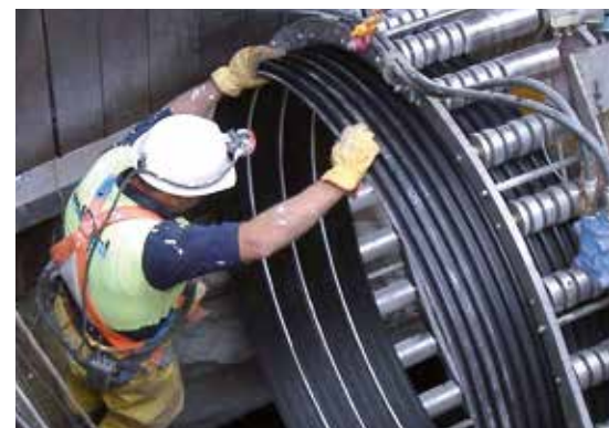
SPR™ PE liner being produced by the winding machine
