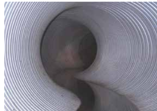
Rehabilitation of bends
