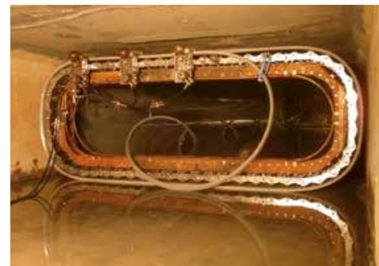
Rehabilitation of custom shape
