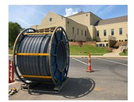
Spiral Wound is a fully structural solution with a limited construction footprint above ground; an appropriate choice for the area. It also allows the contractor to install with flow present in the pipeline. This proved critical as managing the flows became a substantial challenge from the start.
