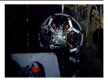
Ruby-Collins completed the 60" portion in May 2020, lining over 1,100 LF of RCP. They immediately transitioned to SPR™TF virtual training and prepared to line the 42" section. With all the delays and the challenge of virtual training, they were able to successfully line the 400 LF section of 42" RCP in June. The combined effort from Kemi Construction, Ruby-Collins Inc, SEKISUI SPR Americas, and Fulton County officials pushed the project to completion.
