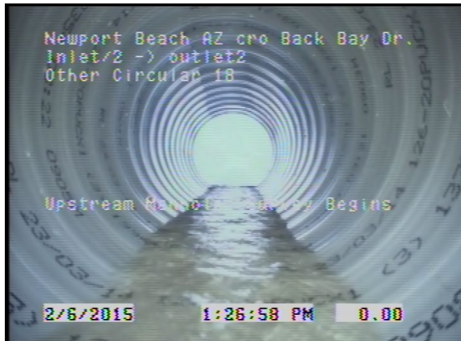
Figure 7. Post Installation Using Spiral Wound Liners
